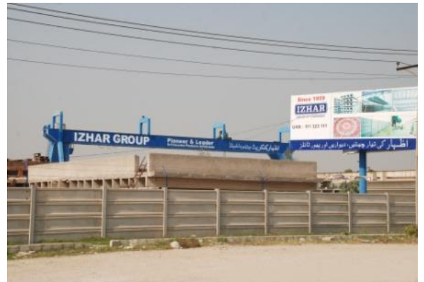
Izhar Concrete Limited GT Road Muridke
