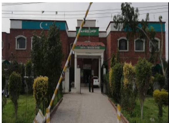
Figure 12: Front view of MC Office Building
