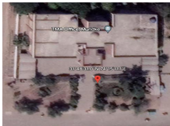
Figure 13: Ariel view of MC Office Buildings
